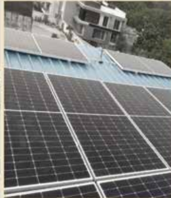
Option III: Shed (South/East-West Facing) Space Needed: 60-70 sq. ft./KW
